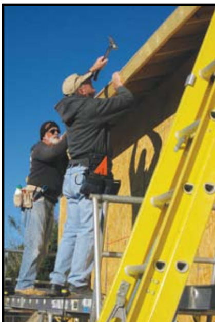
Andy Leatherman (right) hammering on the job for Habitat for Humanity.
